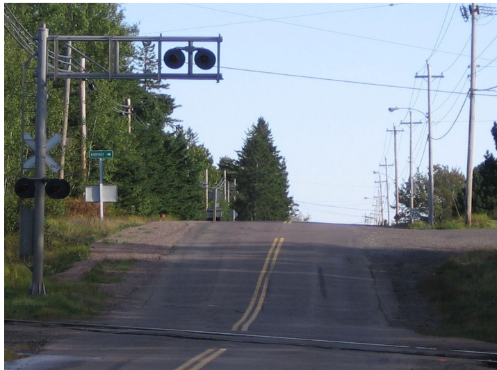
Figure 2: Railway warning signals are often elevated to offer better conspicuity of the crossing at a distance. In this example, the signals have been elevated to compensate for poor visibility of the level crossing due to vertical curvature of the road.
