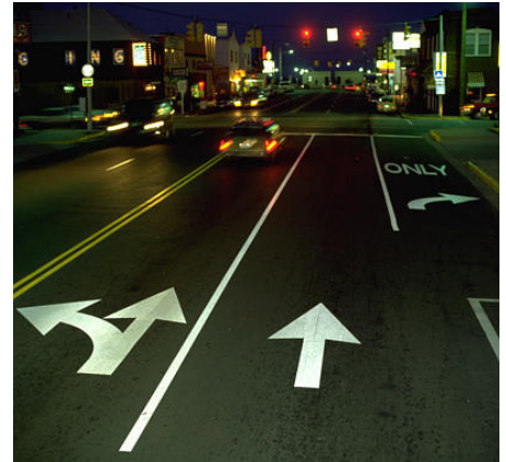
Figure 2: Although this is an urban intersection, the effect of durable pavement markings is still evident. Such a treatment may be employed at rural intersections where it is not possible to provide illumination.
