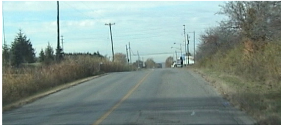
Figure 3: If there are changes in the vertical alignment of a roadway (a steep uphill or steep downhill section), an intersection that is located beyond a crest curve may not be visible to a driver. In regions of the country where the terrain is relatively flat, any change in the vertical alignment near an intersection may be a cause for driver confusion. A higher number of rear-end and right-angle collisions may occur at intersections where a vertical curve is located on the approach.
