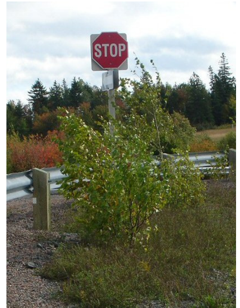
Figure 1: Roadside shrubbery has been allowed to grow to a height at which it now threatens to obscure the Stop sign. It already obscures sight lines. Poor maintenance such as this presents a significant risk to drivers.
