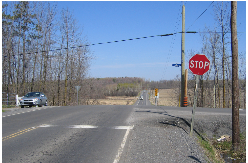
Figure 1: This three-legged intersection has Stop or Yield signs on each leg. Caution must be given to permitting such applications. If all-way controls cannot be defended by warrants, they should not be used. Note: the Yield sign is inappropriately applied in this situation.
