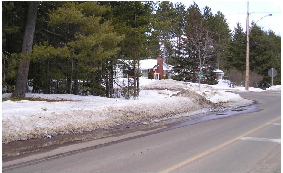
Figure 3: The presence of trees has reduced the sight distance to approaching vehicles at this intersection. While the problem is not notable in this photograph, snow accumulation can also be a significant cause of poor visibility at intersections.
