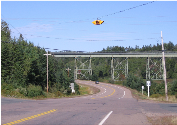
Figure 6: Installation of an overhead flashing hazard beacon above the intersection, visible from all approaches. The overhead beacon should supplement the standard signs and traffic control required at an intersection. This is a commonly used solution, however its effectiveness has not been adequately documented.
