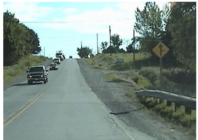
Figure 4: This photo provides an example of the effect that a vertical curve can have on the ability of a driver to see an approaching intersection. A closer look reveals that there are visual clues in the photograph such as platooning vehicles (sometimes indicative) and a warning sign, but the intersection itself is not visible. The combination of a horizontal and vertical curve will tend to make this problem more acute.
