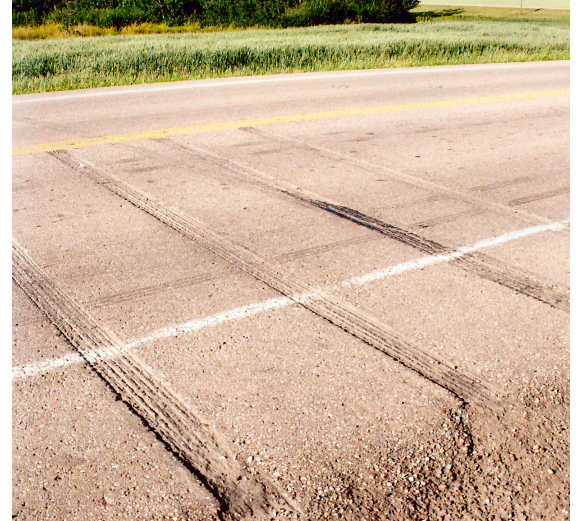
Figure 3: This photo illustrates the use of grooved transverse rumble strips on the approach to an intersection. This type of treatment is appropriate to rural areas where there are no residences nearby as they can be noisy. They are sometimes used on long stretches of roadway such as in the prairies when the intersection is not readily apparent, or where there is a history of "Running Stop Sign" crashes.
