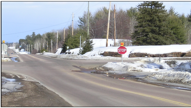
Figure 5: Flashing beacons may be used to supplement signs, as shown in the photo. Be aware that numerous warning signs on the approach to an intersection may distract or confuse a driver. Care must be taken to install an appropriate number of warning signs in the correct location on the approach to an intersection.
