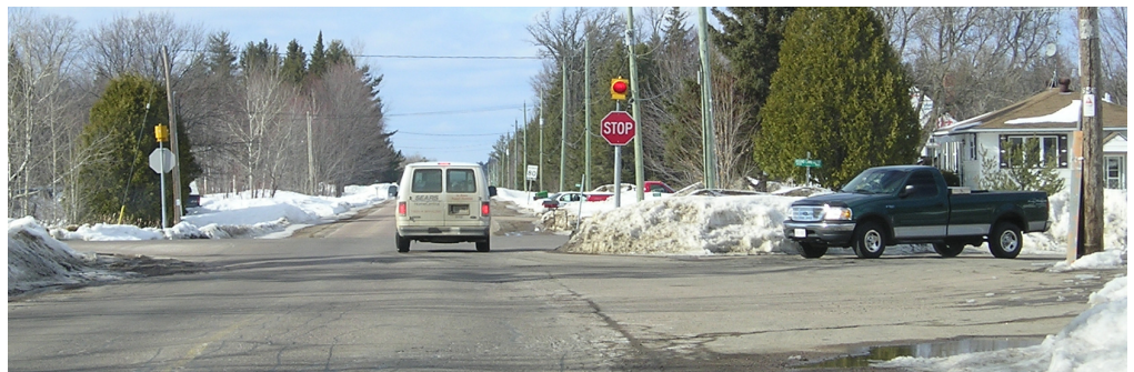
Figure 1: In this situation, the commercial entrance in advance of the intersection results in increased driver confusion in determining where to come to a stop or to turn. Compensation has been provided by adding a flashing beacon over the Stop sign. Better lane markings could also be provided, but the best solution is to reduce and relocate the driveway.
