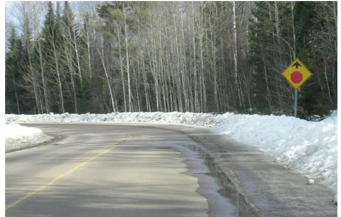
Figure 1: Example of a horizontal curve to the left where an Advance Warning sign has been erected to compensate for poor visibility around the curve.
