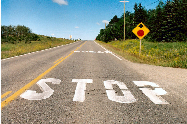
Figure 2: While there are no data to demonstrate their effectiveness, the use of words on the pavement in support of signage is a legitimate application. Note how the sign and pavement markings work to reinforce one another. Section D of the MUTCDC contains the appropriate specifications for the use of words on pavements. This example is from Alberta.
