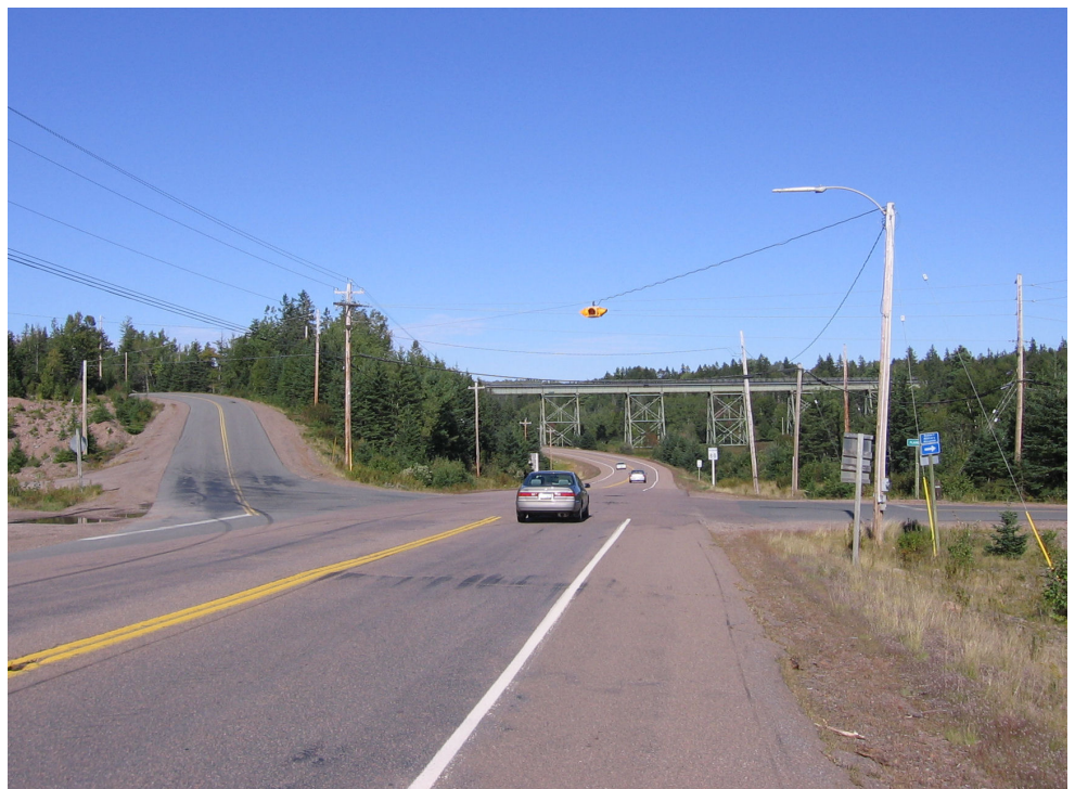
Figure 1: Roads that intersect at sharp angles can create problems for large turning vehicles and they extend the length of time and distance that is needed to enter or cross the intersecting road. The photograph shows a skewed intersection with the minor road in the left of the photograph. In this example, there is an unusual additional problem with the minor roadway in that it could be confused with the through travel path of the major road. This section offers solutions to problems such as these.
