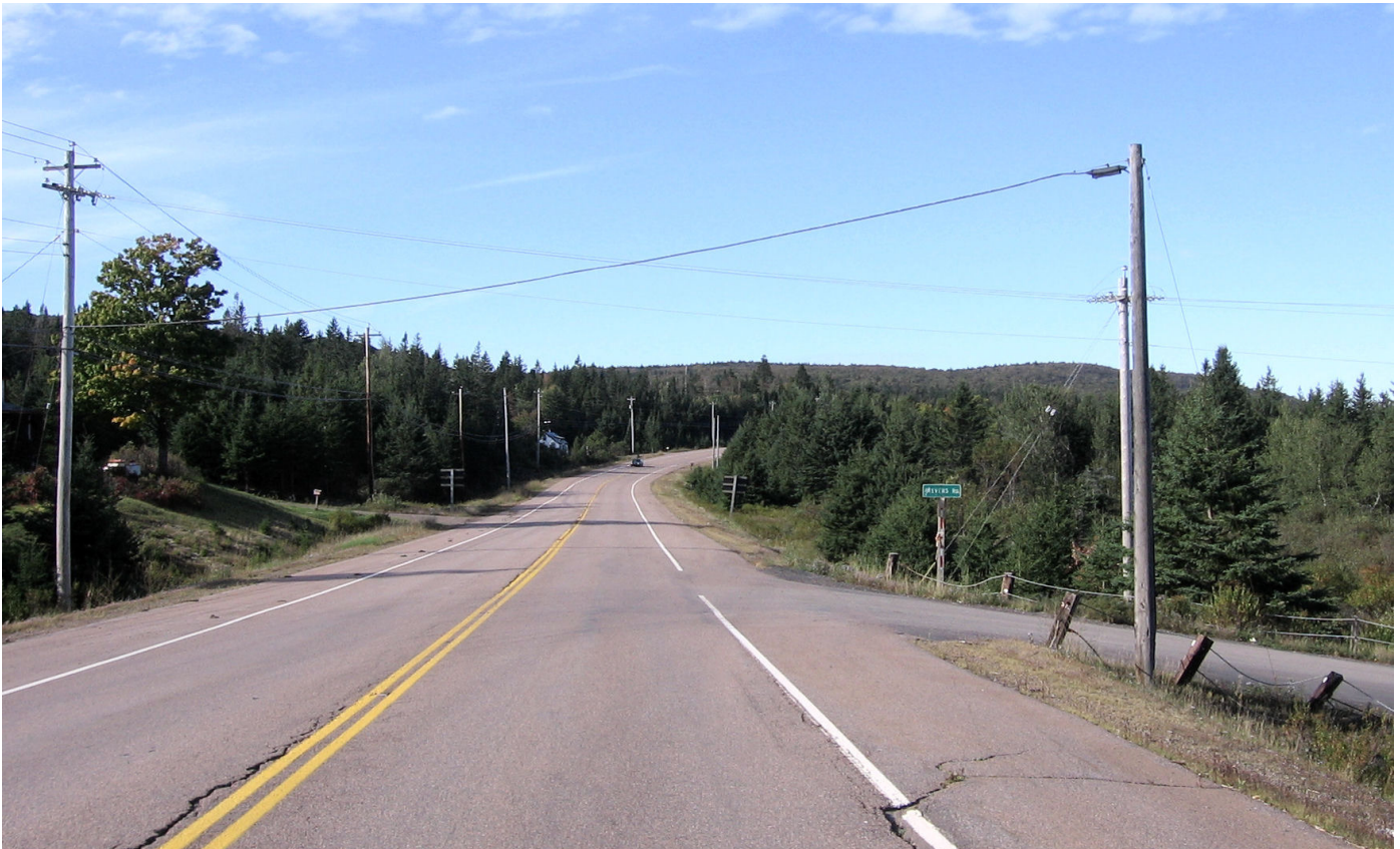
Figure 2: Utility poles present a significant hazard to drivers when located too close to the travel lane as in this example. Note also the poorly maintained cable barrier on the right.
