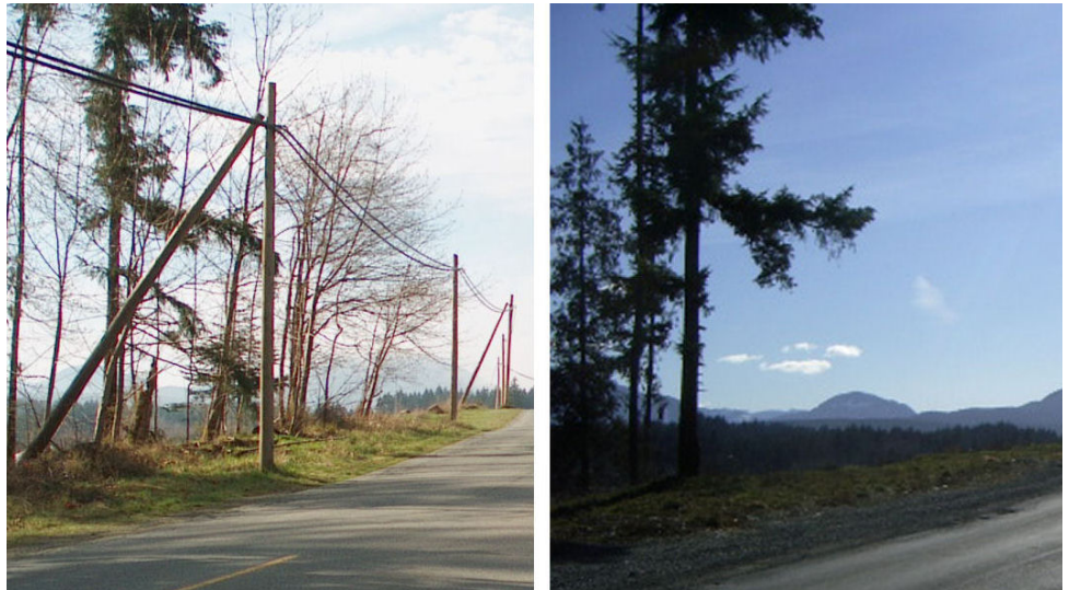
Figure 1: Utility poles can present a significant hazard to drivers encroaching on the roadside. In this set of before and after photos, utility poles located adjacent to the roadway have been removed to provide an obstacle free recovery zone for errant vehicles. Source: City of Port Alberni.
