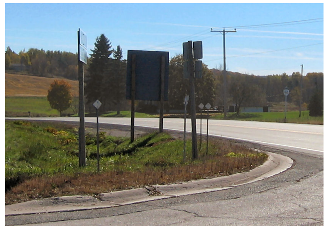
Figure 3: In this variation on sign clutter, this group of signs near the intersection creates a potential visibility problem for turning vehicles that would be particularly acute in winter when snow banks would reduce the low angle view (see also 2.1 Intersection Sight Distance).
