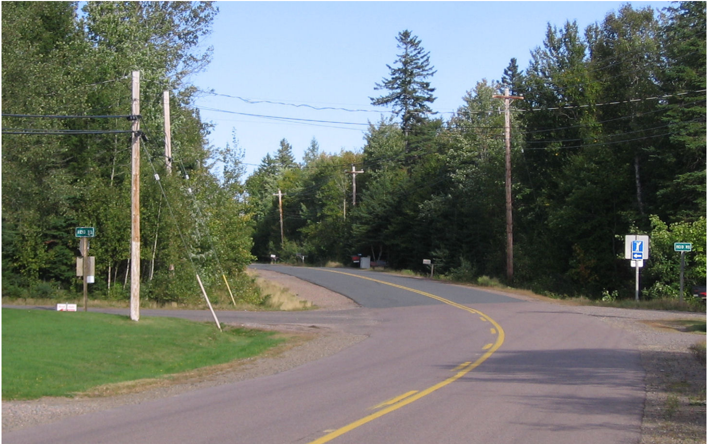
Figure 1: The intersecting road is located on the inside of a curve and there is vegetation near the road. The situation offers very poor visibility, particularly for left-turning traffic from the minor leg. To improve overall visibility and stopping sight distance on the major road, vegetation should be cut back to enable passing drivers time to see the exiting traffic. Also note the lane striping on the major road, which is continuous through the intersection. Proper practice is to break the markings as they pass through an intersection.
