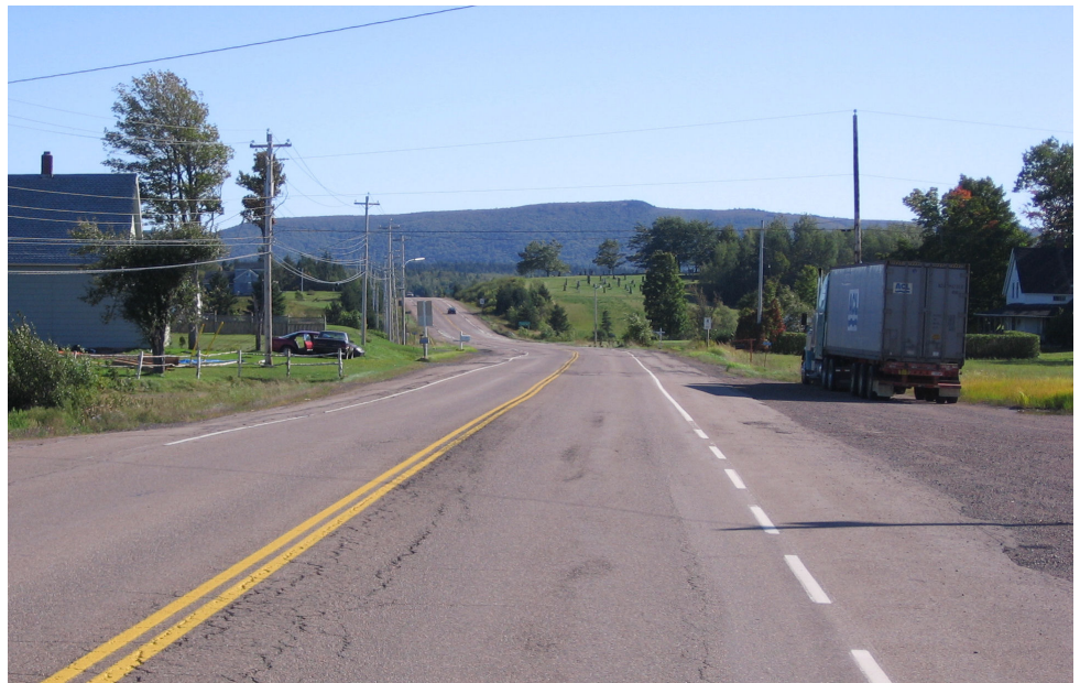
Figure 1: Incorrect use of road markings is as problematic as inadequate road markings. In this example, a skip dash has been applied between the travel lane and the shoulder to signify the presence of a rest stop, however it appears like a passing lane. Following MUTCDC guidelines, the proper application in this case would be a solid line. A sign would be used to denote the rest stop.
