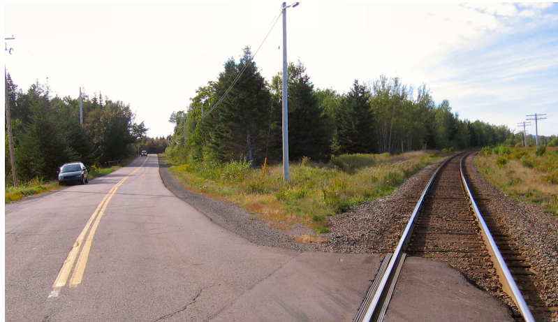
Figure 1: Rail level crossing at extreme angle to the road. Note the clear sightline area.
