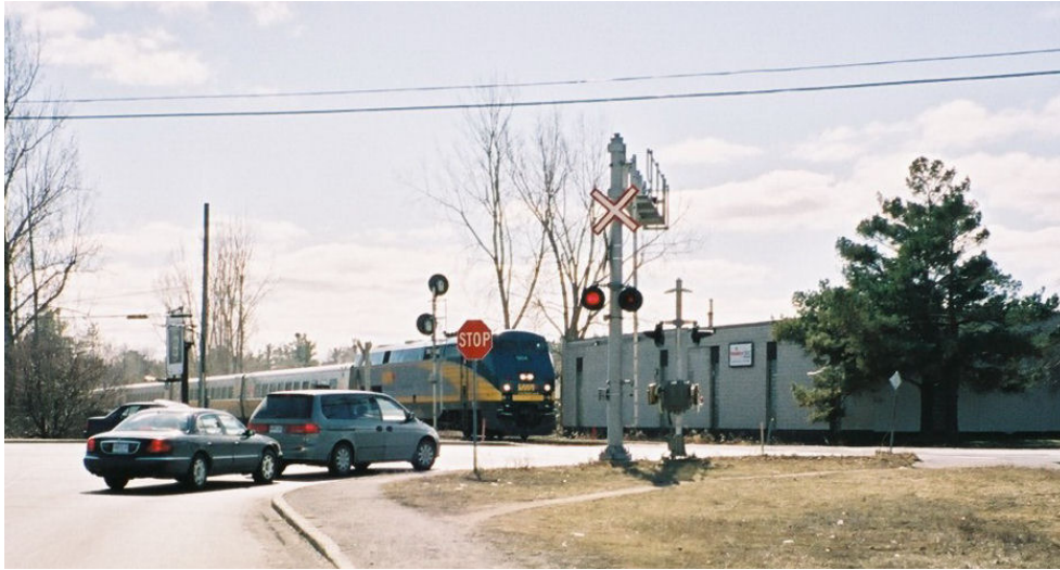
Figure 4: Intersections located in close proximity to a rail; crossing can cause significant road safety and operational concerns.
