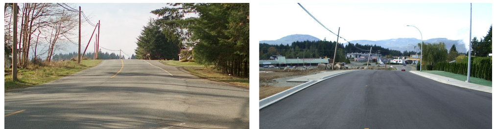
Figure 2: Reduction in vertical curve to improve stopping sight distance. Left: Before; Right: After. Source: City of Port Alberni.
