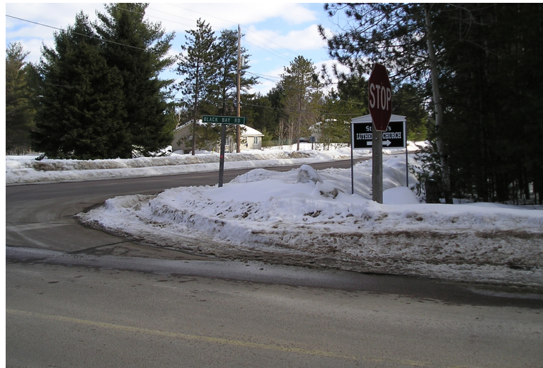
Figure 2: The signs in this photo have obstructed the sight distance for vehicles waiting to enter the intersection.
