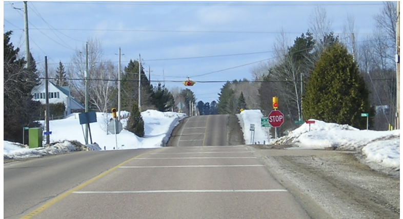
Figure 7: Another application of an overhead flashing beacon with the addition of supplementary transverse pavement markings (optical speed bars) on the intersection approach. Use these with caution, as these markings become faded and worn and may not be visible in wintertime.
